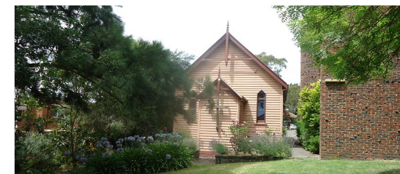
P3. EXISTING TIMBER CHURCH.
